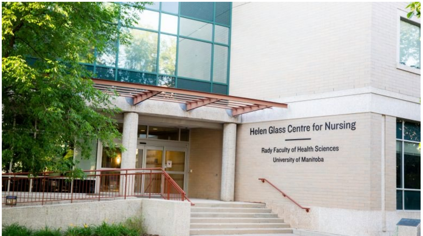
Helen Glass Centre for Nursing 89 Curry Place Front entrance view
